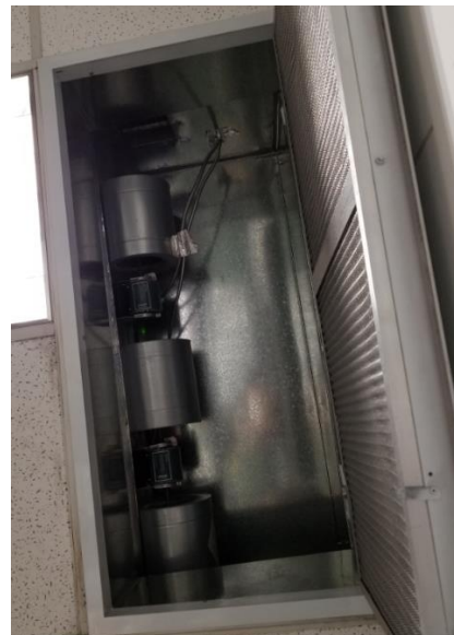
Photo 5 – Installed PMSM
