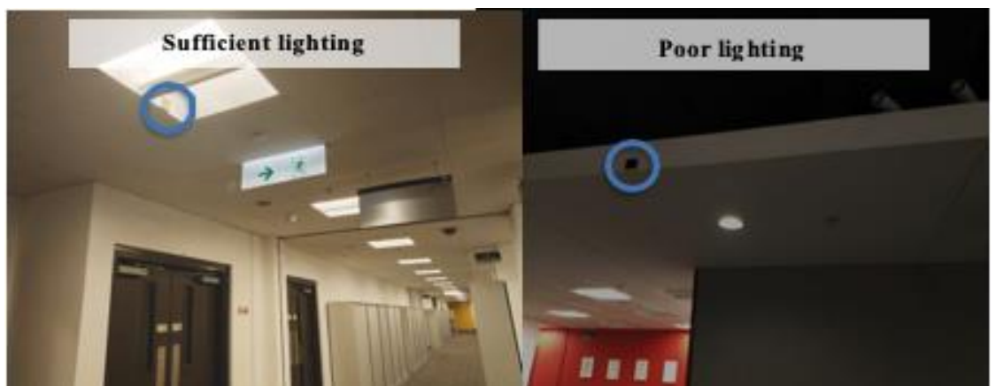
Fig 3. luXbeacons deployment locations with varying lighting conditions on 6/F and 7/F of the EMSD HQ.
