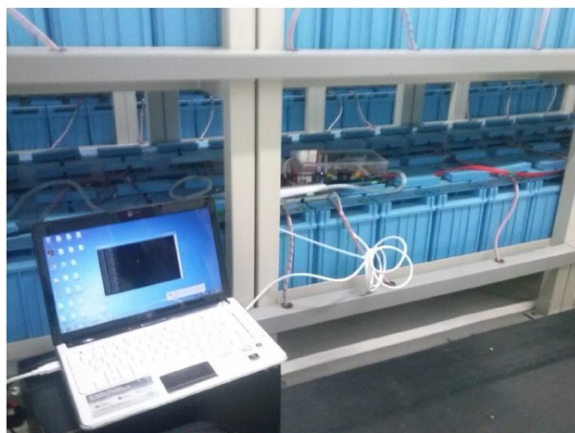
Smart Real-time Battery State and Health Diagnostics System at Siu Ho Wan Data Center
